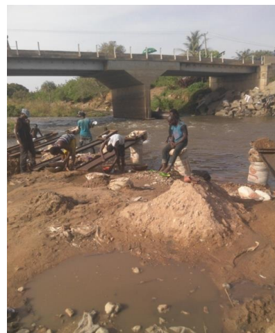
Fig. 6: Shows some artisanal miners carrying out sluicing process at the Manyara river
